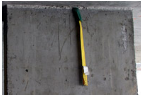
Figure 2 - In-deck anchor set in column
