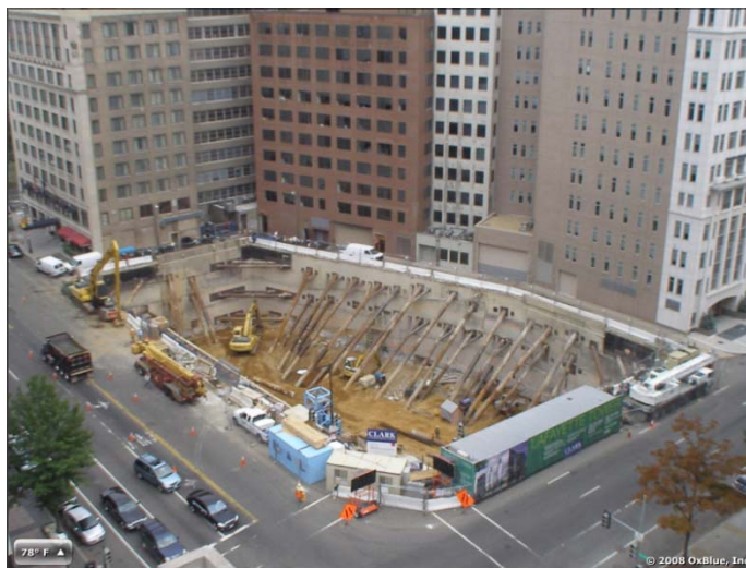
Figure 1 - Lafayette Tower during demolition of the existing structure
